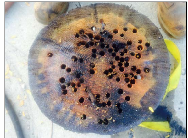
Pier 3 pile cross-section showing marine borer damage
