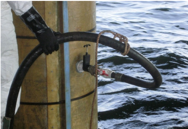
Preventative maintenance repair
