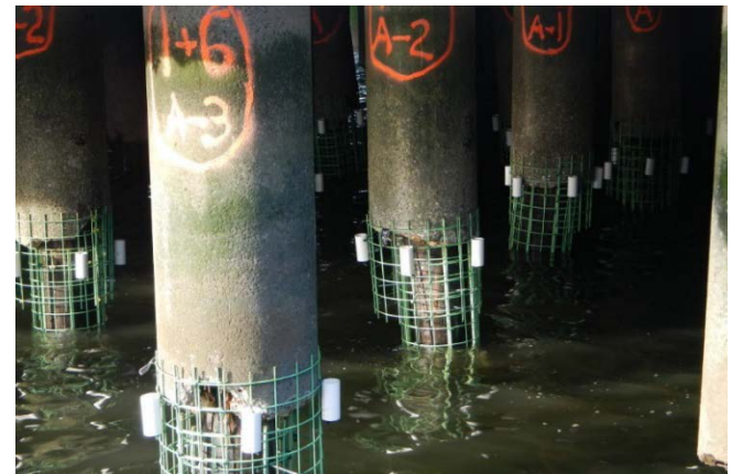
Reactive maintenance pile repair
